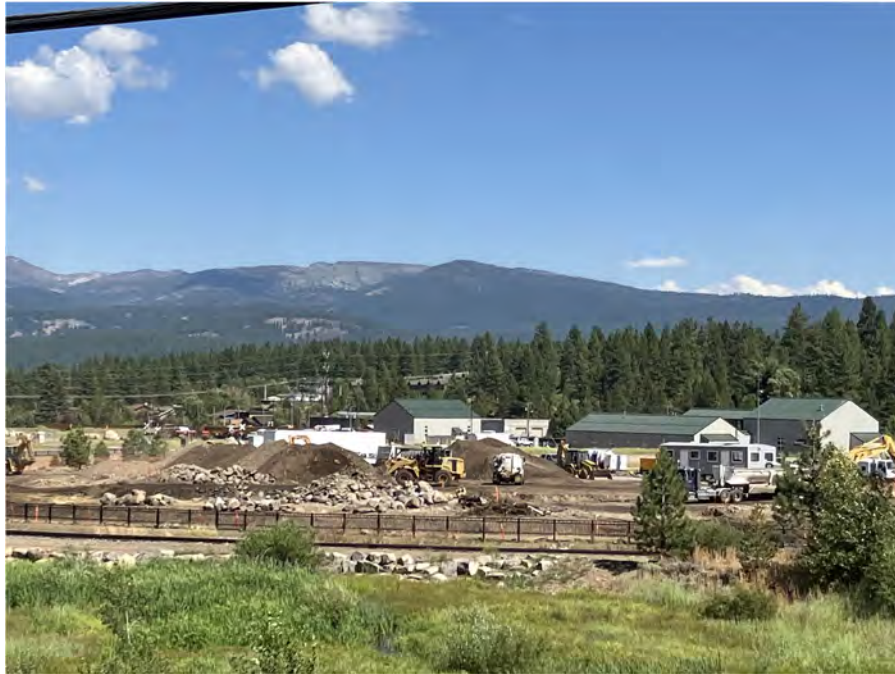
Figure 3: Early Construction, August 3, 2023
